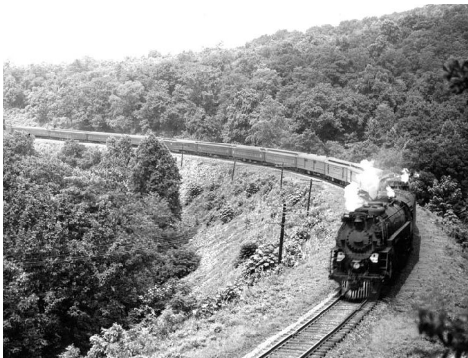
J-3 No. 606 and J-3A 610 pull a heavy train near Little Rock Tunnel in July 1949. When passenger trains exceeded 14 cars, a helper was required. (J. I. Kelly Photo, C&OHS Collection, COHS 316)
