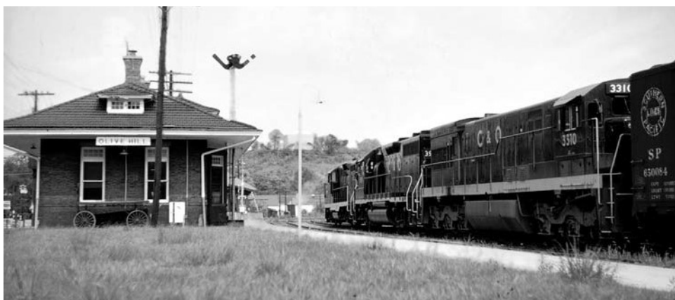
Eastbound "switcher" is stopped at Olive Hill depot, in August 1969 while crew checks out orders inside. This GE (1968) U30C diesel has GSC 3-axle trucks. Many C&O's U30C's had trucks designed by Adirondack Steel Castings. (Eugene L. Huddleston Photo, C&OHS Collection, COHS 23720)
