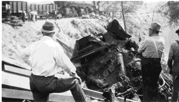
The wreck of westward freight Train 73 at Gulfco, Ky., May 29, 1935. K-3a Mikado No. 2313 was hauling 28 cars and a caboose; the engineer and lead brakeman were killed. (C&O Historical Society Photo Collection, cohs-80022)
