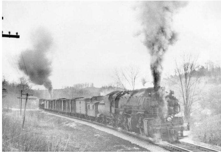
An eastbound freight climbs the 2.66 percent grade near Mountain Top, Ky., ca. 1950, with an H-6 2-6-6-2 pusher from Olive Hill backing up behind it — about to cut off on the fly at the summit, as described above. Photo by Gene Huddleston. (C&O Historical Society Photo Collection, cobs-21065)
