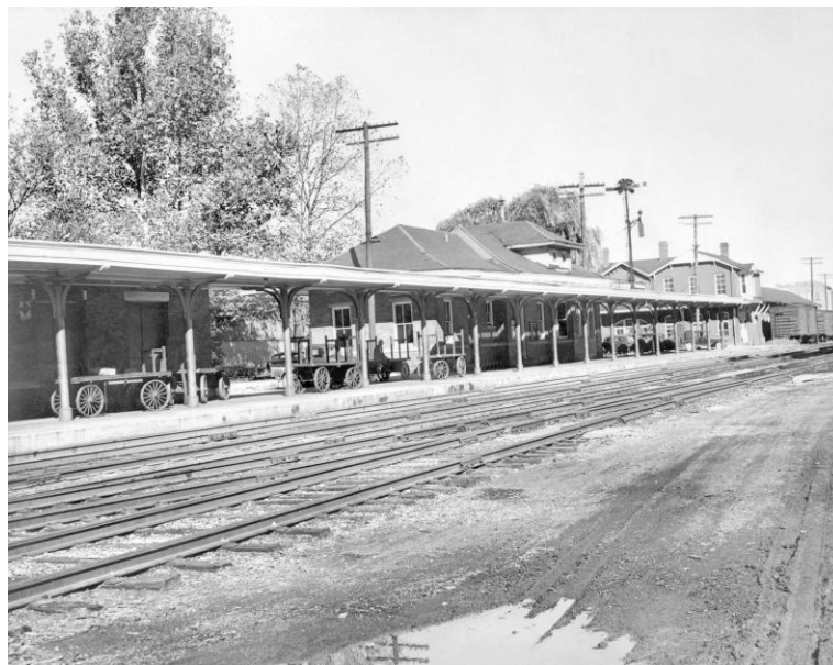
The C&O passenger station at Mt. Sterling, Ky., looking east, showing the platform canopy and the two-story brick freight station behind it, ca. 1944. (C&O Historical Society Photo Collection, cobs-21471)
