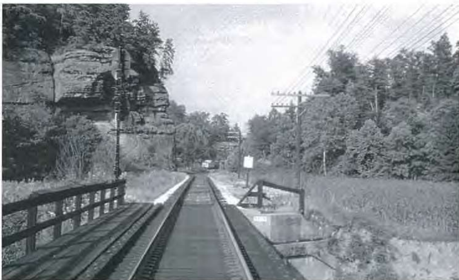
A 1958 view, facing east toward the area of the 1961 washout at Aden. The cliff at left was subsequently blasted away by the Army Corps of Engineers as part of flood-control efforts.
