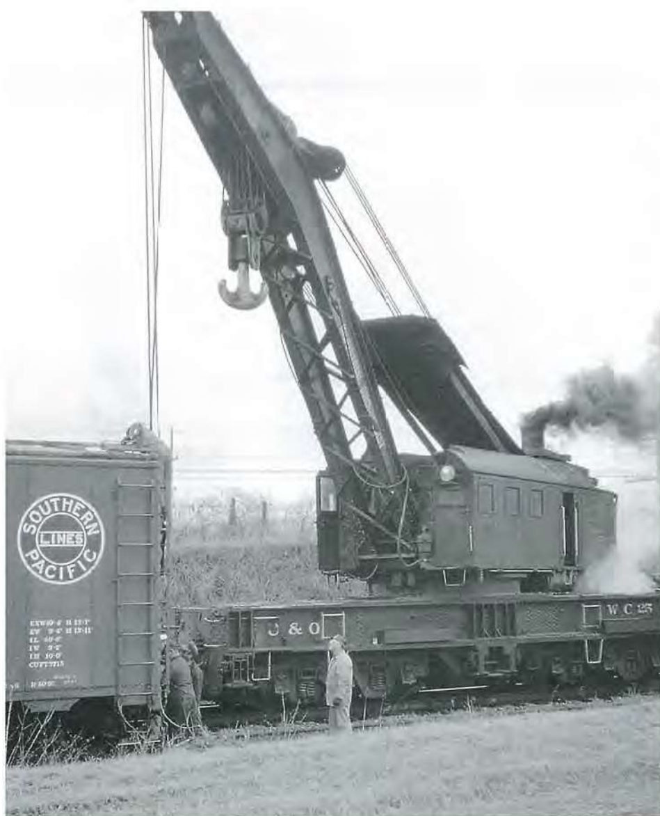
C&O 250-ton wrecker No. WC-25 worked near Limeville, Ky., in March 1963. (Don Riel)
